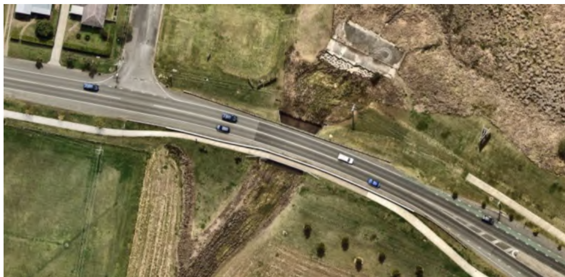
Figure 20: Bridge Crossing on Albert Street near Boundary Street
