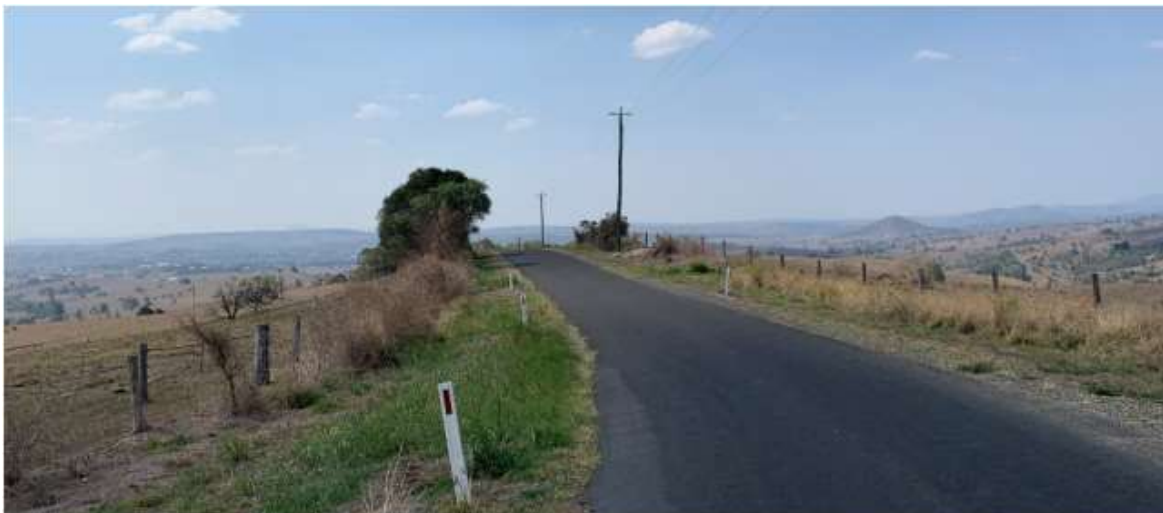
Figure 2: Site Inspection Photo
