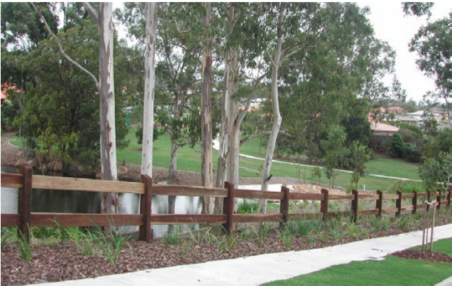
Open post and rail timber fencing to mark lot boundaries but still allow for flow of water when required
