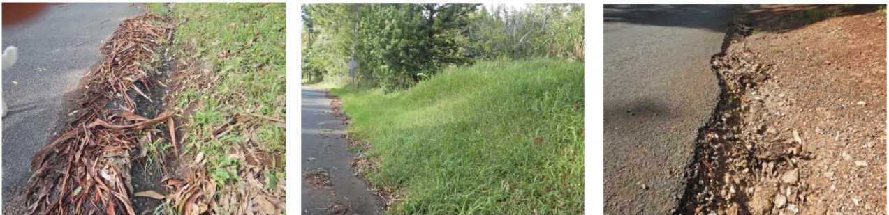
Washed out gutter. Overgrown Gutter & uncut grass inviting snakes & vermin. Washed out gutter near 93 Long Road, near roundabout.
