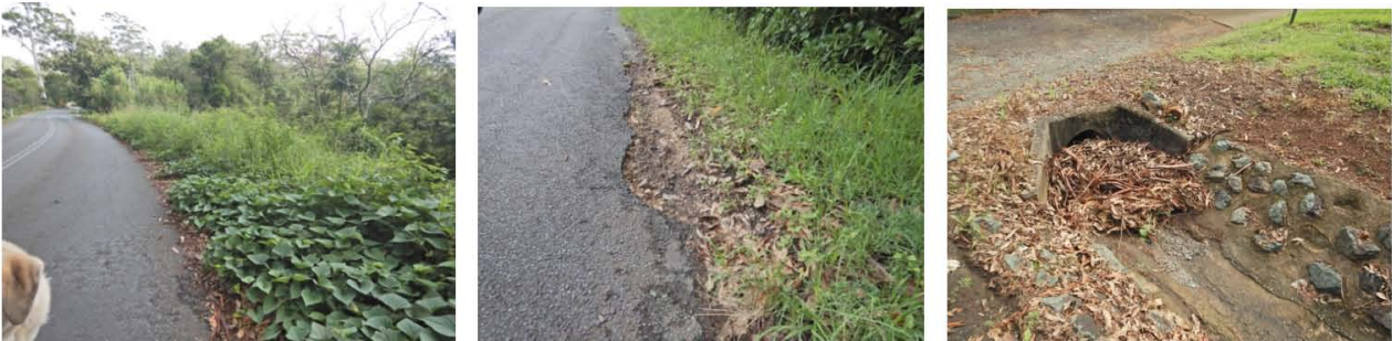
Overgrown weeds along the road north of Katoomba Court. Washed out & eroded gutter eastern side of road. Blocked drain outside 62 Long Road house will cause major problems with more rain.
